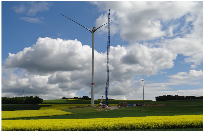
Erection of the wind park Bärweiler
